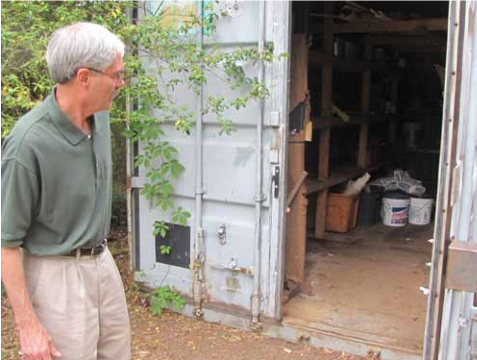
The vandalized DeKalb County Habitat for Humanity sheds are filled with tools again thanks to donations from White Cap and the Atlanta GSC.
